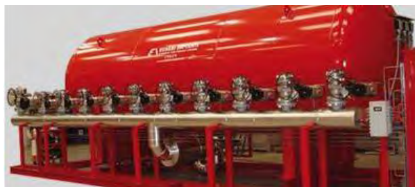
Isothermal modules with CO 2 (liquid firefighting gas unit)
